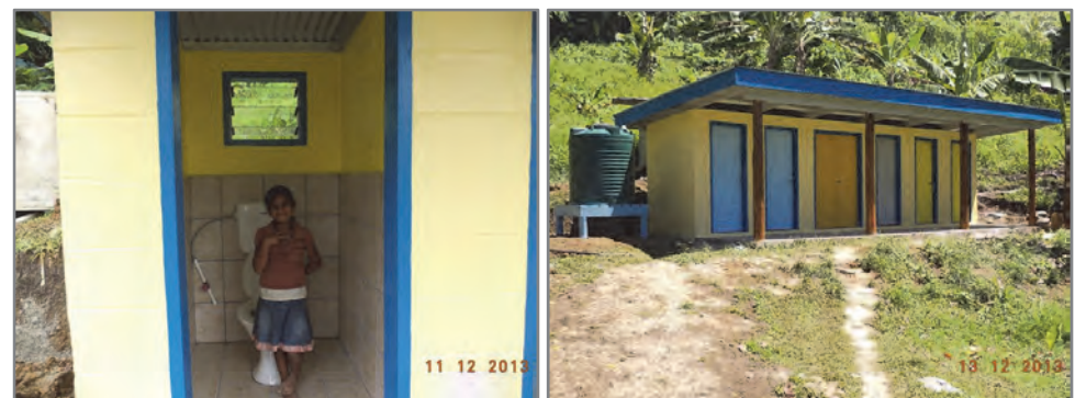
The completed toilet and drinking block
